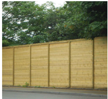
4m High Acoustic Fence
